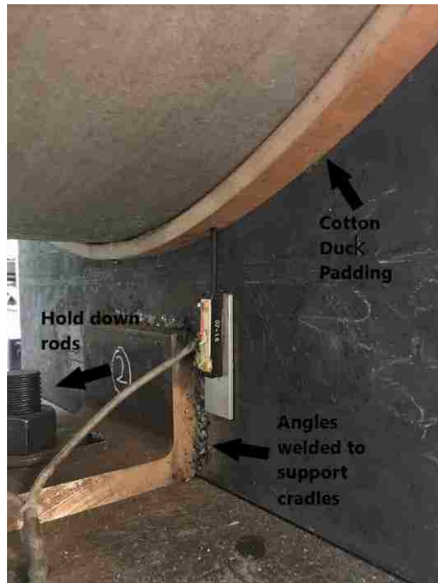
Figure 3-21. Support cradle arrangement
