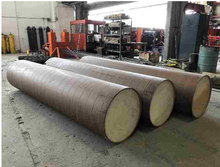
Figure 3-9. Sonovoid® round concrete void forms
