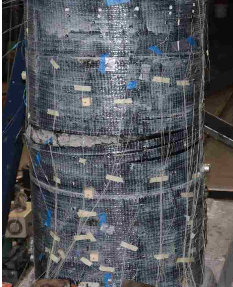
Figure 7-14. Fiber rupture on north face during Series 11
