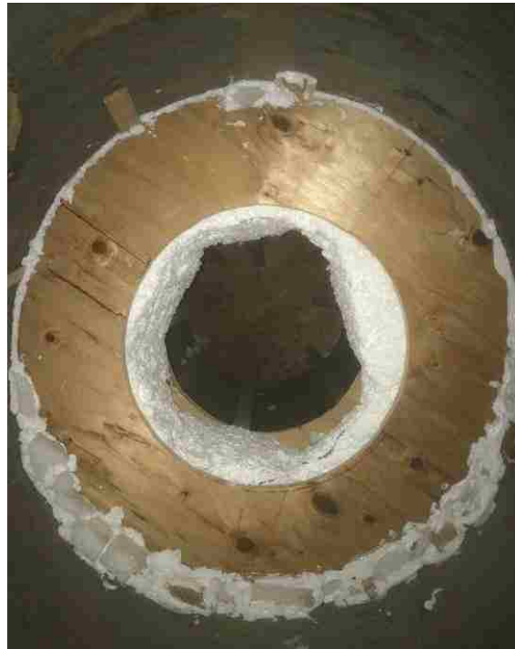
Figure 3-15. Foam spacer followed by last plywood ring
