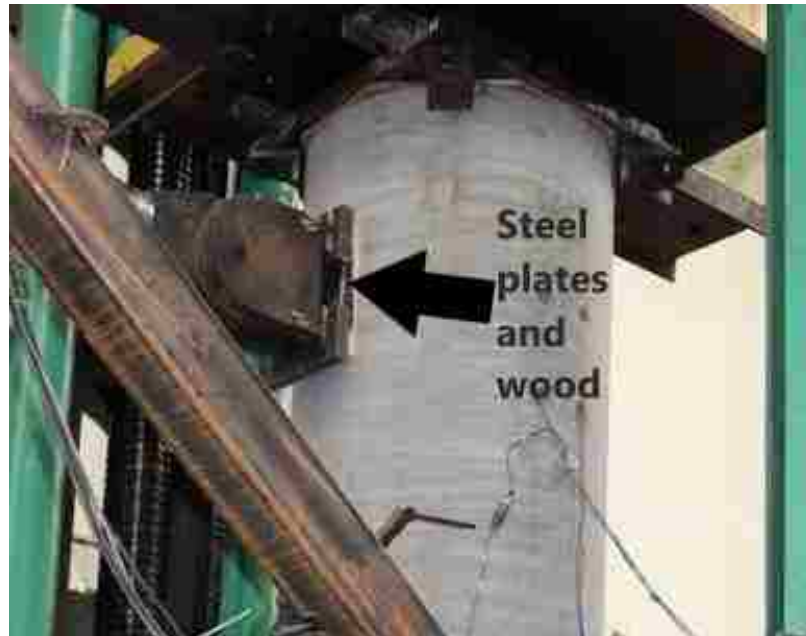
Figure 8-4. Packing underneath actuator connected to specimen
