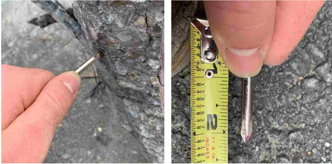
Figure 7-23. Measuring of the strand slip
