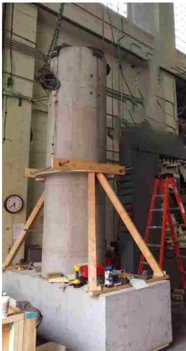
Figure 6-15. Pile-column braced on top of cap beam
