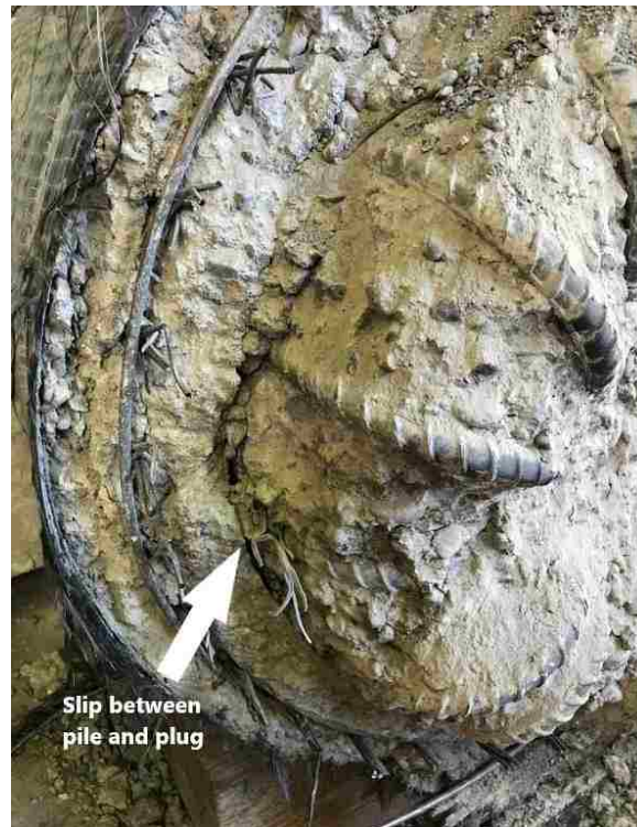
Figure 7-18. Looking down at plug reinforcement after top segment of specimen (portion above the plug in test orientation) had been removed
