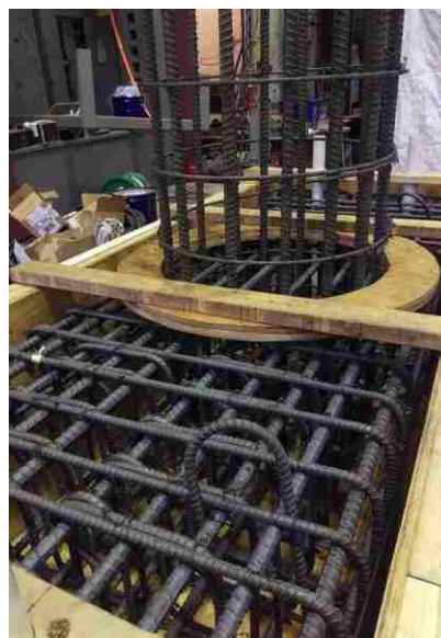
Figure 6-12. Cap beam and plug reinforcement in formwork before casting
