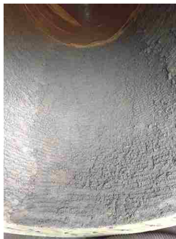
Figure 6-14. Inner surface of pile-column roughened with epoxy mortar
